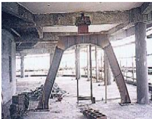
Figure 7 Construction site of LVD
