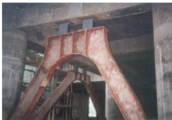
Figure 9 Construction site of LVD
