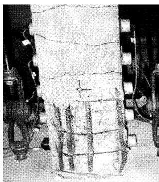
Figure 3: Insufficient transverse reinforcement in the plastic hinge zone and the subsequent extensive damage to the pier (Saadatmanesh et.al. (1997))
