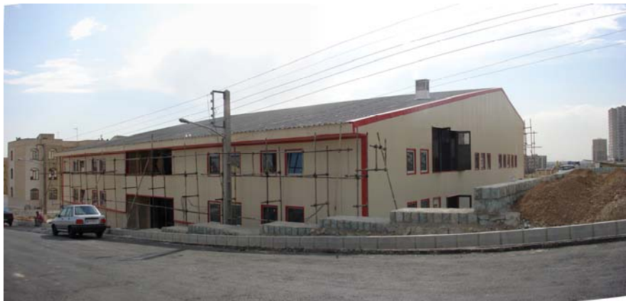
Figure 5 One of the Disaster Management Bases constructed in Tehran
