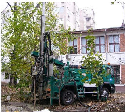
Figure 8 Drilling equipment on truck
