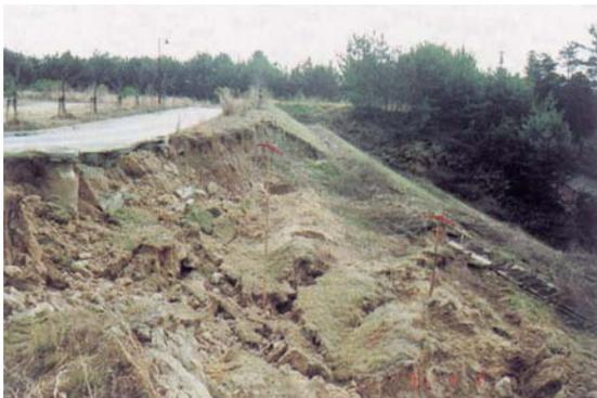
Figure 9 Slope failure due to 2001 Geiyo Earthquake shock
