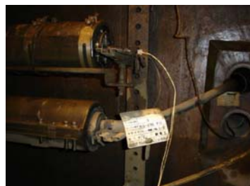
Cable cut in manhole The Niigata Chuetsu Earthquake
