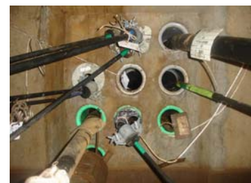
Cable displacement in manhole Niigata Chuetsu-oki Earthquake
