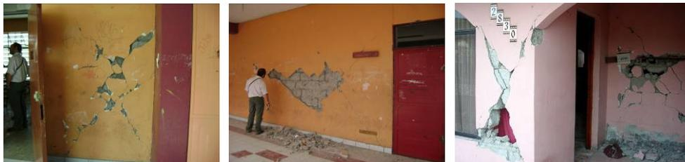
Figure 1 Damages due to in-plane shear action in Chilean masonry buildings, Tocopilla earthquake ( $M_w=7.7$ ), 2007.
