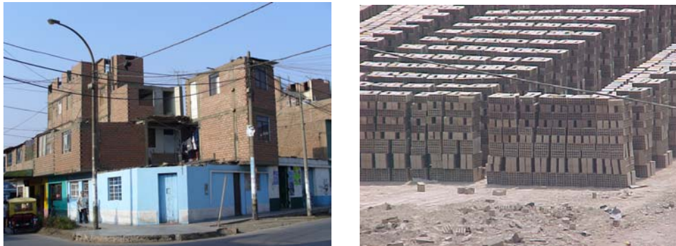
Figure 1. Left: buildings with tubular-masonry bricks. Right: Storage of tubular-masonry bricks in unconventional factory.
