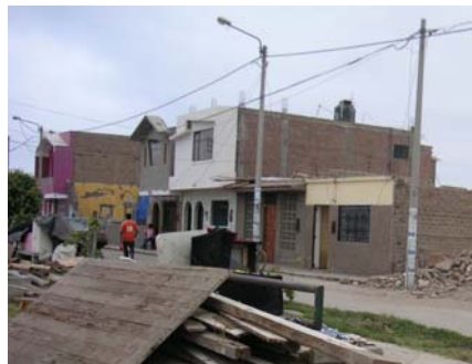
Figure 12. 2-story tubular masonry wall buildings in Pisco, without damage. Regular configuration.
