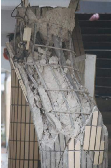
Fig. 1. Failure of a reinforced concrete column caused by inadequate flexural ductility
