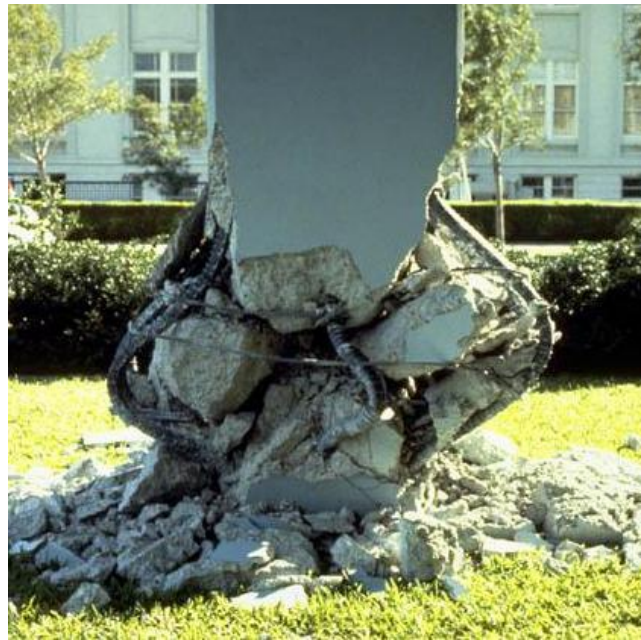
Fig. 2. Shear failure and migration of plastic hinge region
