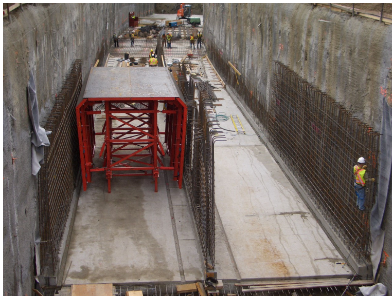
Figure 6 Side-by-side Box Steel Form and Wall Reinforcing
