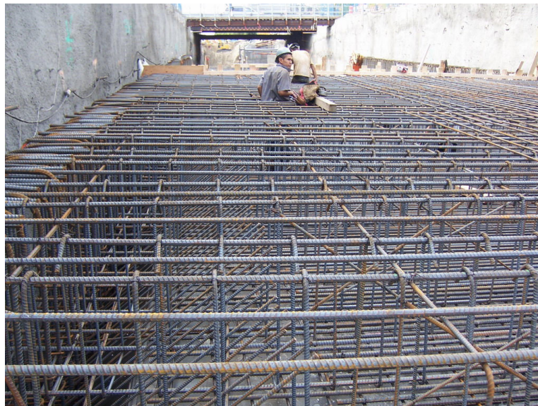
Figure 8 Roof Slab and Wall Reinforcing
