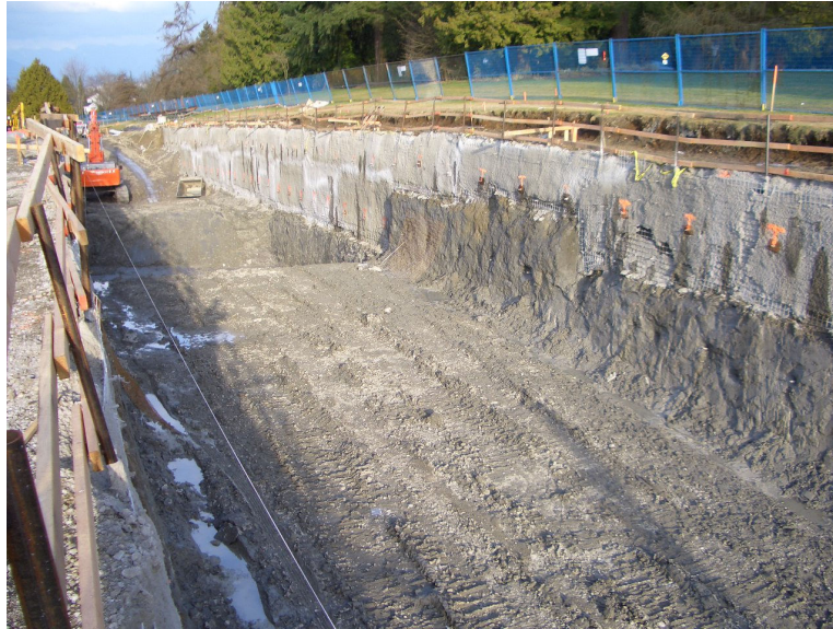
Figure 5 Excavated Trench near Little Mountain
