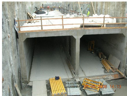
Figure 7 Roof Slab of Side-by-Side Box
