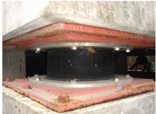
Photo 2. High-damping rubber isolator
