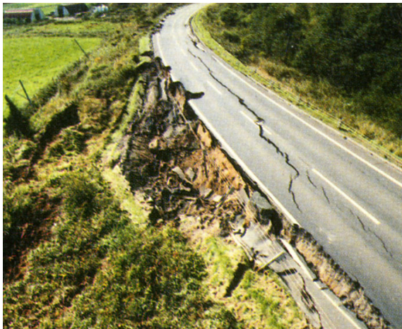
Figure1 National highway embankment damage in the HOKKAIDO TOUHOU-OKI Earthquake
