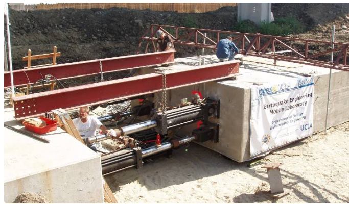
Figure 3: Nine pile group specimen before testing
