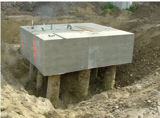
Figure 10: Group specimen after soil excavation
