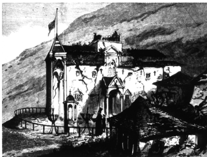
Figure 2. Main church damaged at Atalanti due to the 1894 events, drawn from a sketch by W. C. Bourchier (Albini & Pantosti 2004)
