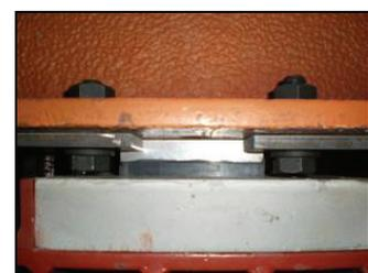
Figure 6 Installation of bearing
