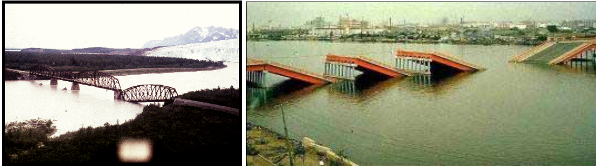
Figure 3: Failure of bridges during earthquakes; (a): Million Dollar Bridge during the 1964 Alaska earthquake (b): Failure of the Showa Bridge after the 1964 Niigata Earthquake. Photo courtesy [21].
