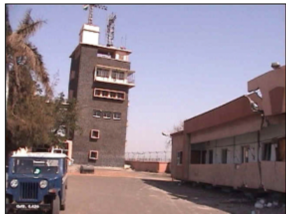
Figure 2(a): Failure of pile foundation in level grounds, after the 1995 Kobe earthquake, Tokimatsu [19]; (b): Collapse of piled Kandla Tower in laterally spreading ground after the 2001 Bhuj Earthquake, Madabhushi et al [20].
