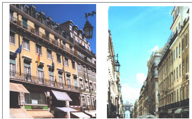
Figure 15 - Introduction of more stories in the top of the buildings (each building has different number of stories)
