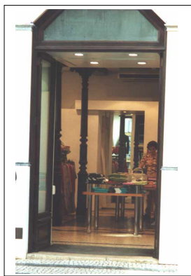
Figure 14 – Metallic element replacing demolished wall
