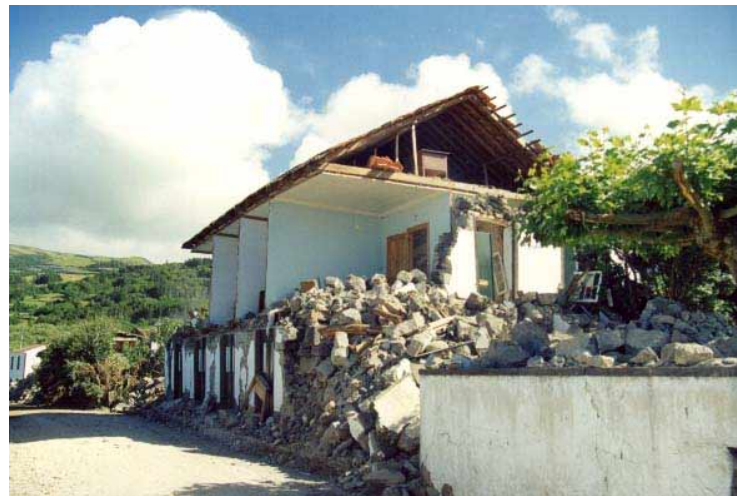
Figure 12 - Fall out the plane of exterior walls without complete collapse (1998 Azores earthquake)
