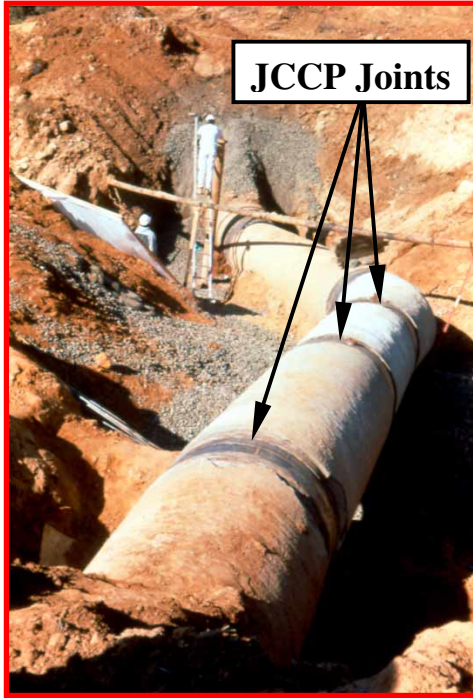
Figure 3 JCCP and Joints (Photo by D. Ballantyne)
