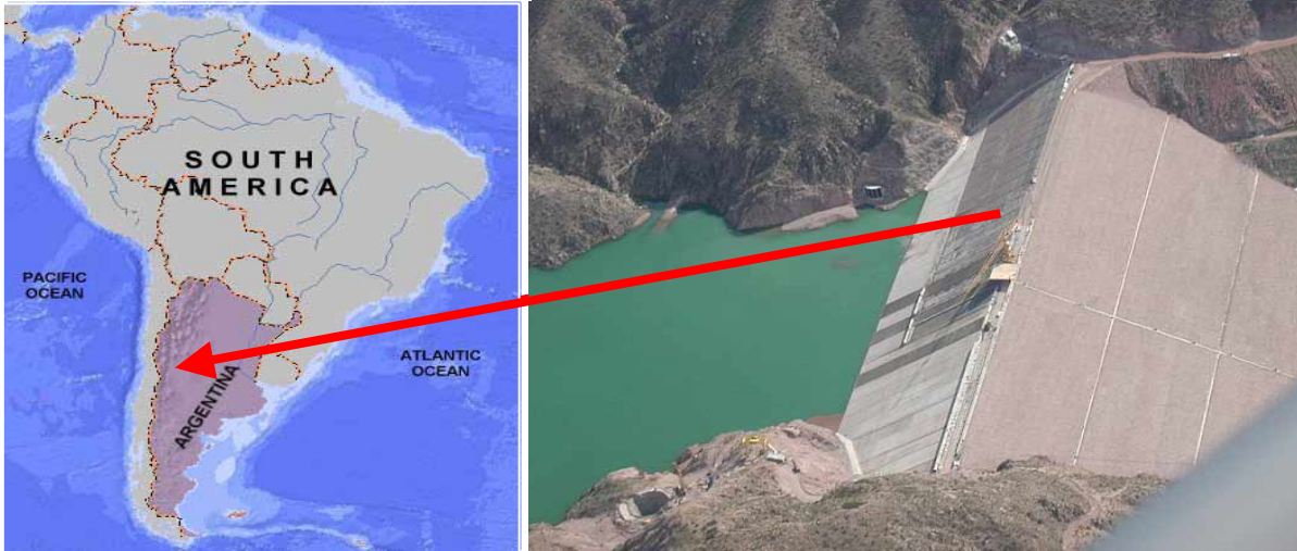
Figure 1- C.F.G.D. Potrerillos Dam on the Mendoza River , Argentina
