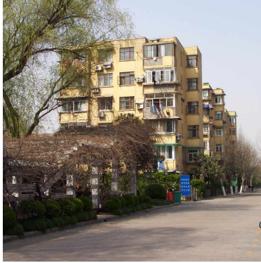
Photo 1. Apartment Building: Type 79-02, Six-storied Building, Tongji Village, Tongji University Campus, Shanghai, China.
