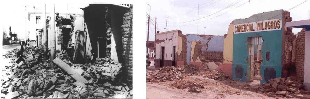
Fig.1. Collapse of traditional adobe houses due to severe earthquakes in Peru.
