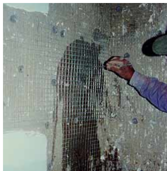
Fig. 3. Sequence of reinforcement on an existing house: Remove the existing cover and perforate the wall (left), connector wire and wire mesh installation (middle), and final cover (right).
