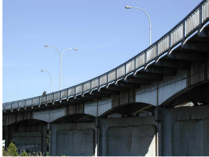
Figure 2 South Approach Girders of the Oak Street Bridge
