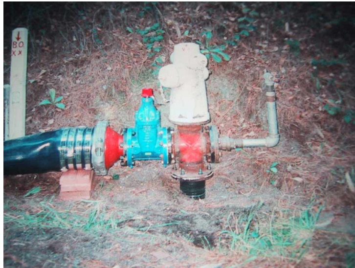
Figure 4. Flex Hose Attachment To Fire Hydrant
