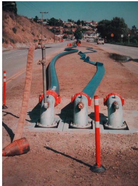
Figure 2. Flex Hose Deployment in EBMUD System
