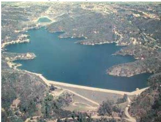
seepage through extensive grouting, the upstream portion of the dam was rebuilt in the mid 1950's. The new portion of the dam was constructed as a roller-compacted earth fill founded on bedrock, but the older downstream portion remained on alluvium. Construction was completed in 1956.
