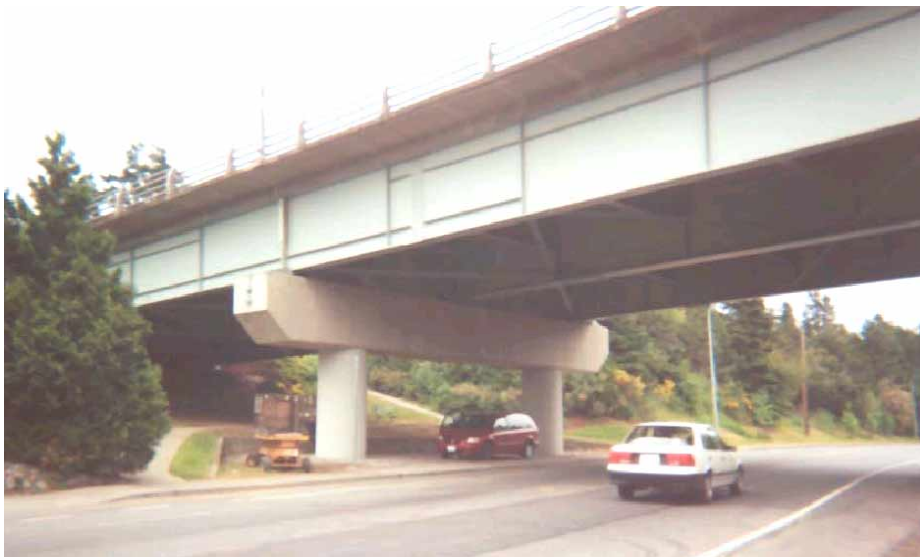
Fig. 1 Portage Creek Bridge in Victoria, British Columbia
