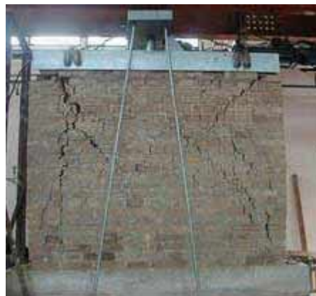
Figure 2. In-plane cyclic loading Test
