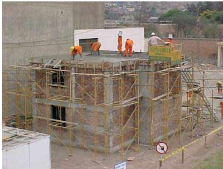
FIGURE 2: The building under construction
