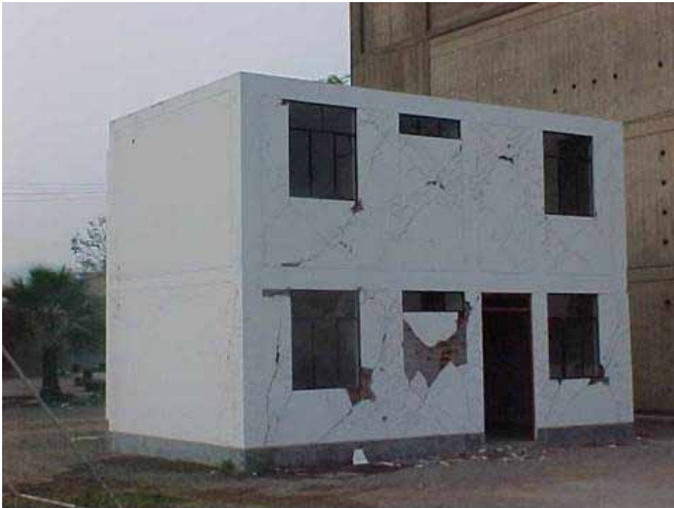
FIGURE 18: South wing of the house in final state
