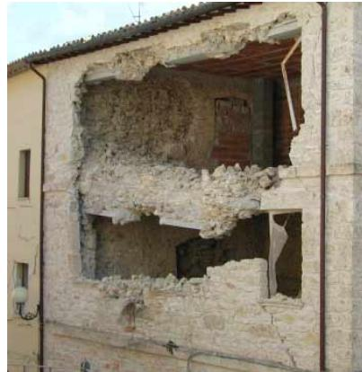
Fig. 2: Rear of the same building were a large overturning of the façade occurred, due to the high percentage of openings, combined with the presence of a heavy r.c. floor supported by poorly connected double-layer masonry.
