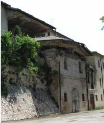
Fig. 1: Collapse of the upper floor of a building due to the substitution of the timber roof with a heavier r.c. and hollow tiles mixed one, supported by poor masonry walls.
