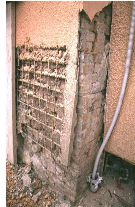
Fig. 3: Loss of effectiveness of a wall strengthened with jacketing to the scarce connection of the steel net through the masonry and the lack of overlapping of the reinforcement at the corners.
