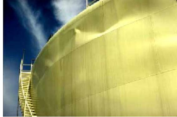
Figures 2.a y 2.b - Earthquake damages of cylindrical storage tanks with flexible shell walls, collection Steinbrugge EERC, U.C Berkeley
