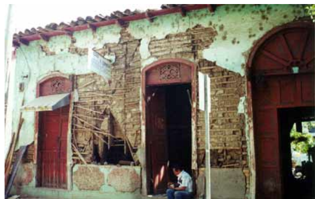
Figure 10. Damage to bahareque in San Vicente caused by the 13 February 2001 earthquake
