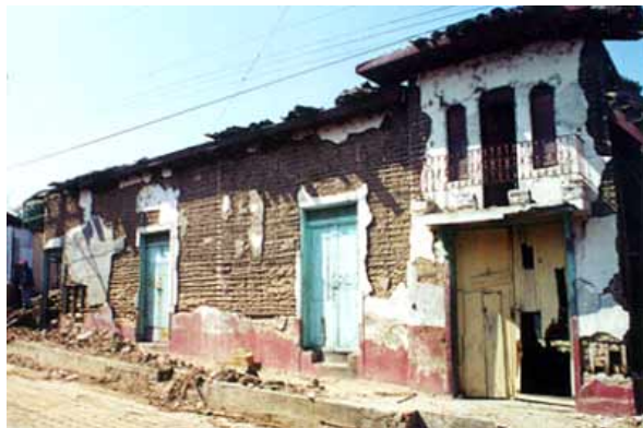
Figure 10. Damage to bahareque in San Vicente caused by the 13 February 2001 earthquake
