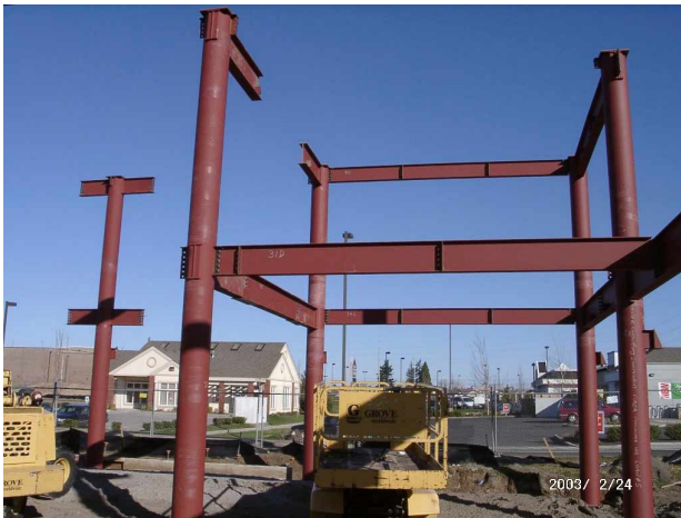
Photo 2a: Shop-fabricated CFT Joint.
