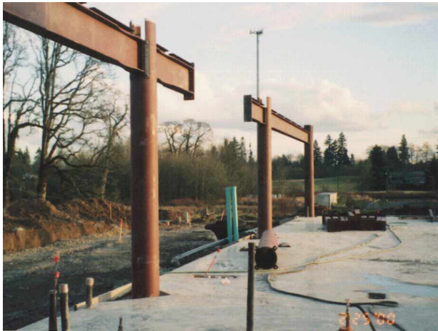
Photo 1a: Field-fabricated CFT Joint.
