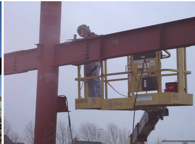
Photo 2b: Girder Connection for Shop Joint.
