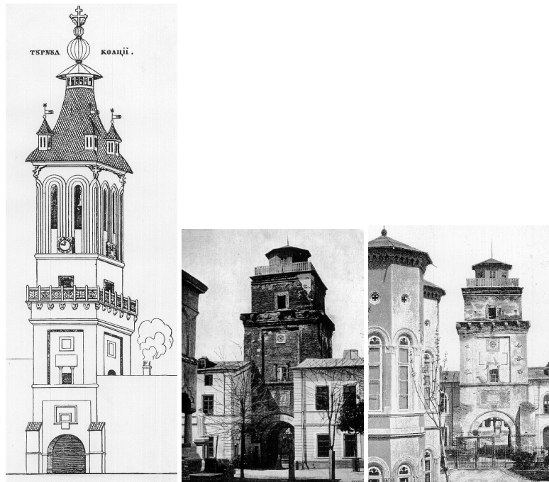
Figure 3. The Coltzea Tower between 1715 and 1802, (Drawing by N. Otetelesanu 1838), (to the left) and the damaged Tower, repaired after 1847, with additional timber stories for firetower, as seen from the East side (middle photo) and West side (right photo) (Photos around 1869, by Carol Popp de Szathmary) [8, 9]
