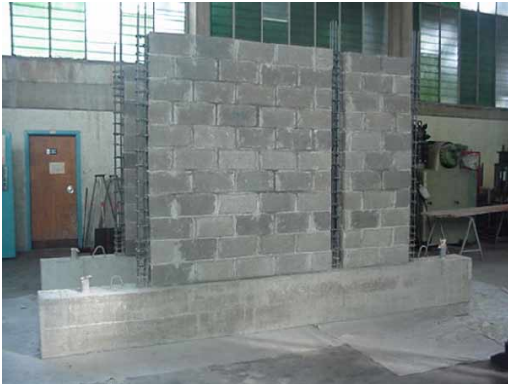
Figure 2. View of the construction process.
