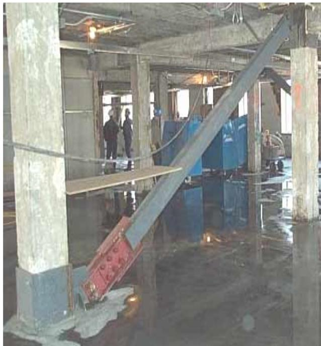
Figure 4. Friction damper at bottom of single diagonal brace
