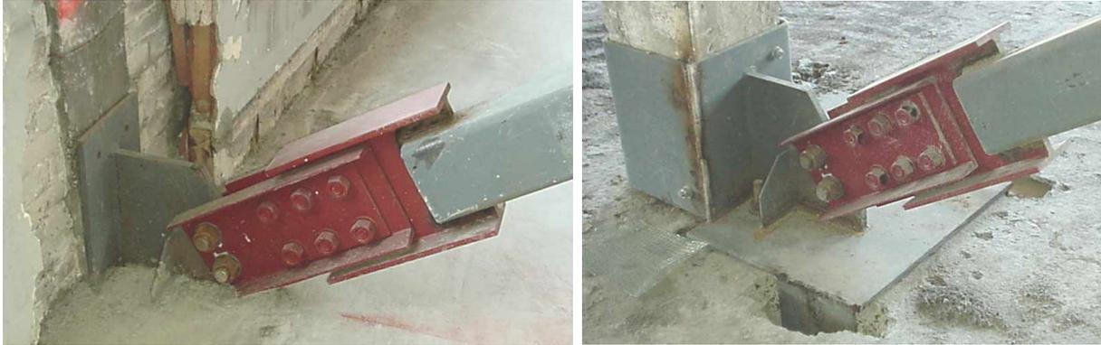
Figure 5. Typical detail of connections
