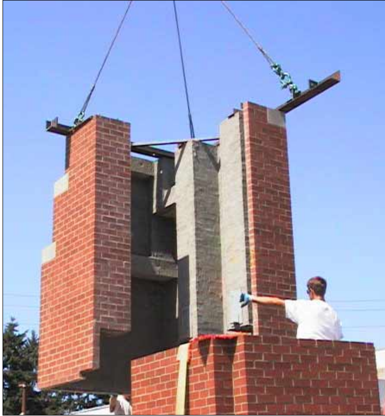
Fig. 10: Reinforced brick corner panel in transit.
