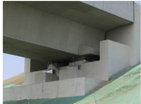
Figure 11: Abutment with extended seating length and special bearings
