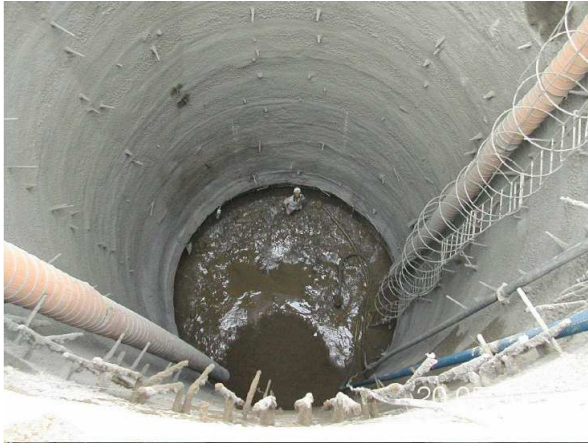
Figure 10: Mono-pile Construction
