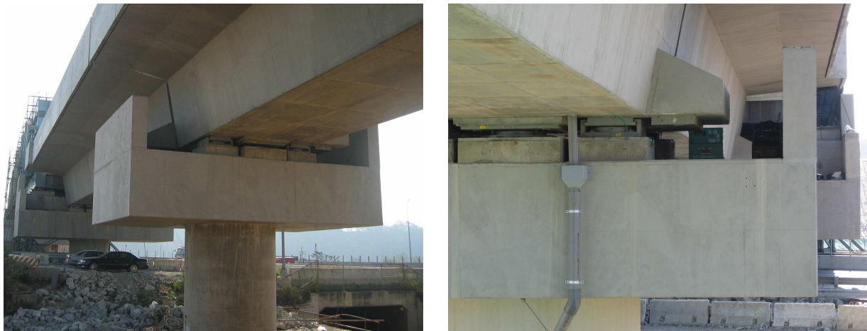
Figure 12: Piers with extended seating length and special bearings
