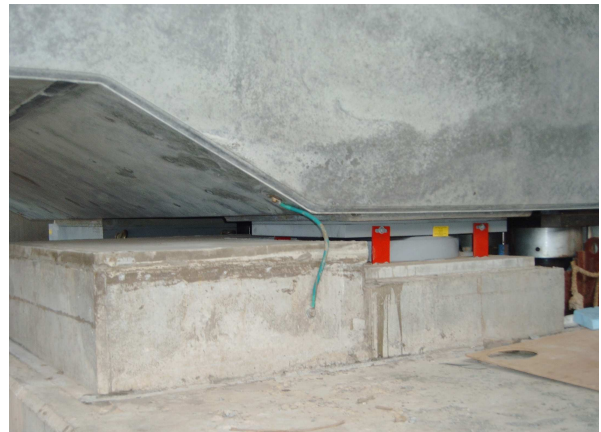
Figure 13: Pot bearings in open mould and on pier caps with sliding surfaces
