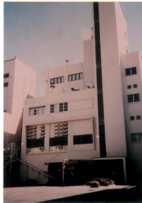
Figure 3: Elevation of the Industrial Building In Van Nuys After Retrofit
