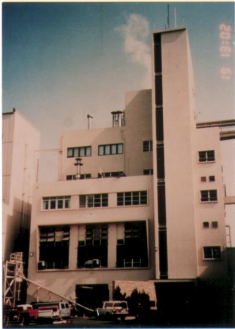
Figure 2: Elevation of the Industrial Building In Van Nuys Before Retrofit
