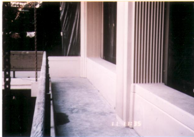
Figure 7: Finished Beams at Second Floor
