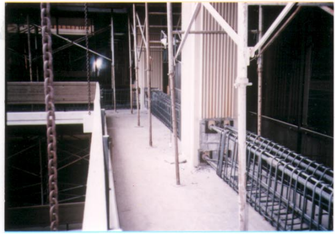
Figure 6. Beam and Joint Reinforcing at Second Level
