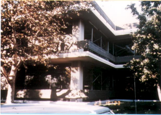
Figure 5. View of Building Exterior
