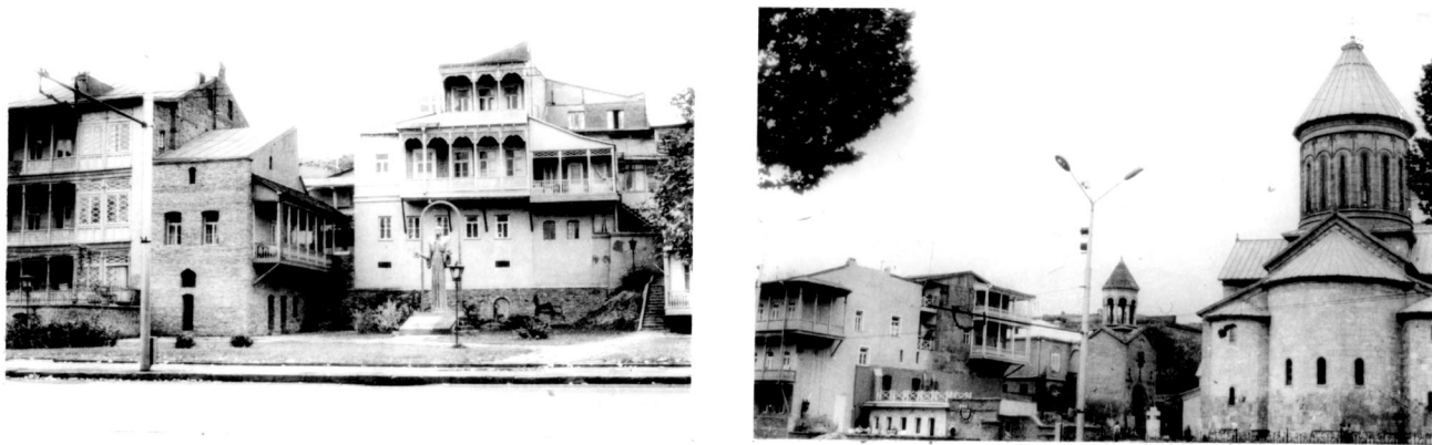
Fig. 2. Reconstruction of the embankment alongside Sioni church.
