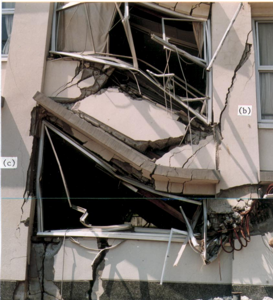
Photo 6 Detail of the third bay
