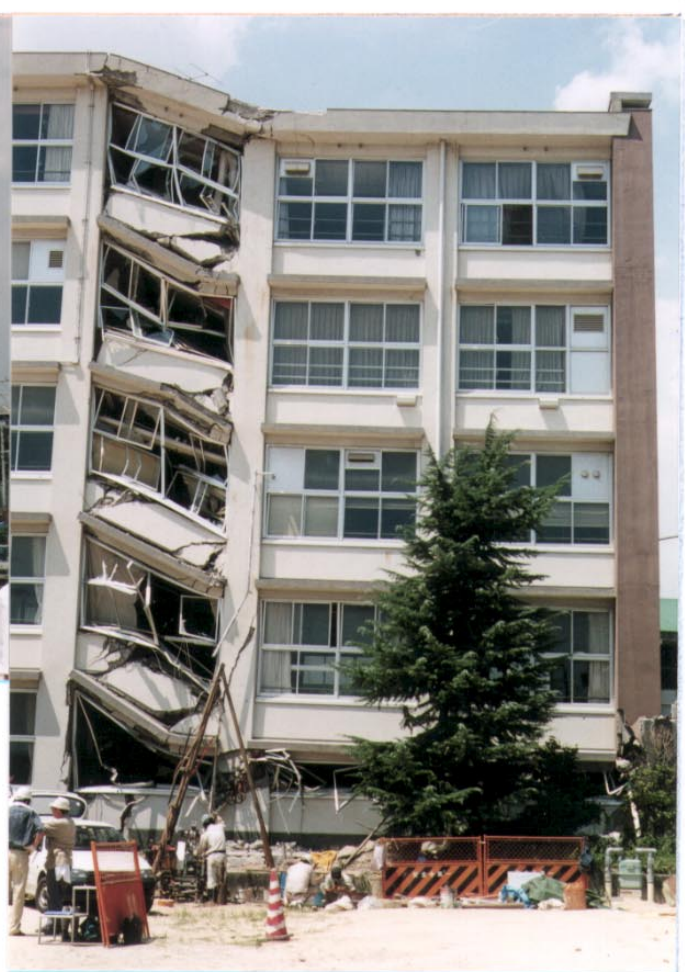
Photo 5 The east two bays
