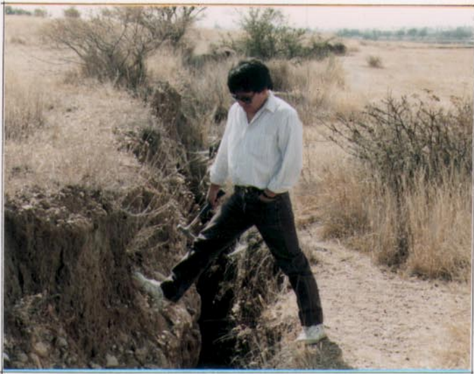
Fig. 2. Fault on the Quaternary sediments (Easter Fault of Aguascalientes). Vertical displacement is of approximately 1 m.
