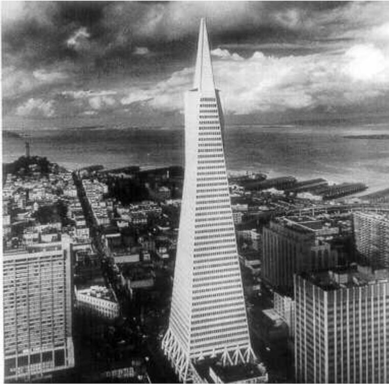
*Though the top floor of the 49-story Transamerica Pyramid swayed more than one foot from side to side in the 1989 San Francisco earthquake, no one was injured nor the building damaged. Casualties were comparatively few in that quake. Most houses that collapsed were built on unstable ground.*
