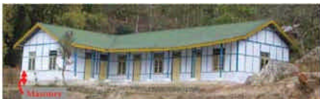
Figure 2. Traditionally constructed typical Ikra structure in Sikkim (school building at Nandok, East Sikkim).
