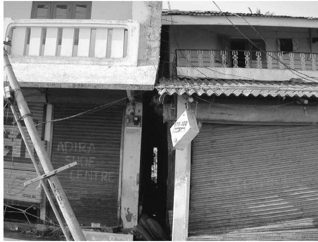
Figure 21. Pounding occurred between closely constructed buildings in and around Port Blair. These buildings are in the Bamboo Flat shopping complex (photo: S. Jain).
