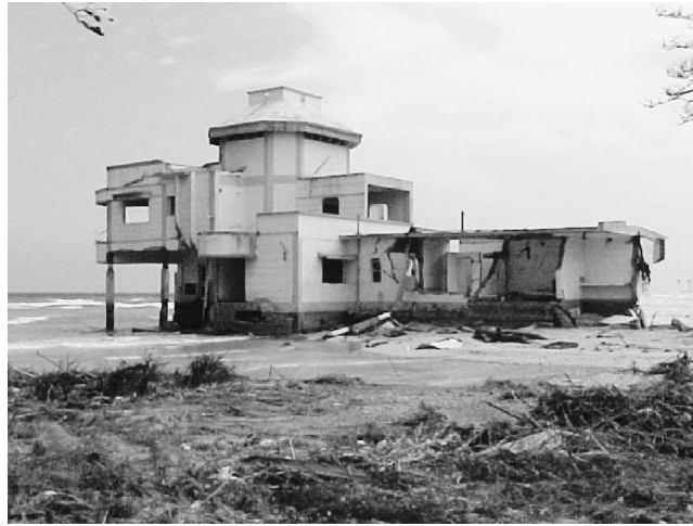
Figure 29. This RC-frame MES inspection bungalow now stands in waters at the Air Force Colony south of Malacca on the east coast of Car Nicobar Island (photo: C. Murty).
