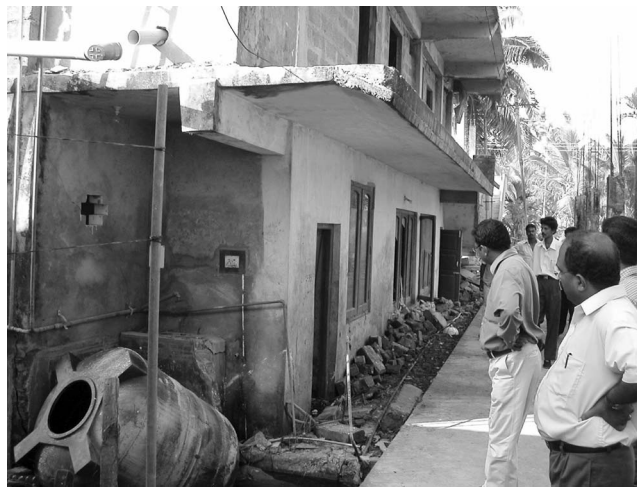
Figure 5. Settlement of RC buildings at Bamboo Flat near Port Blair (photo: H. Kaushik).
