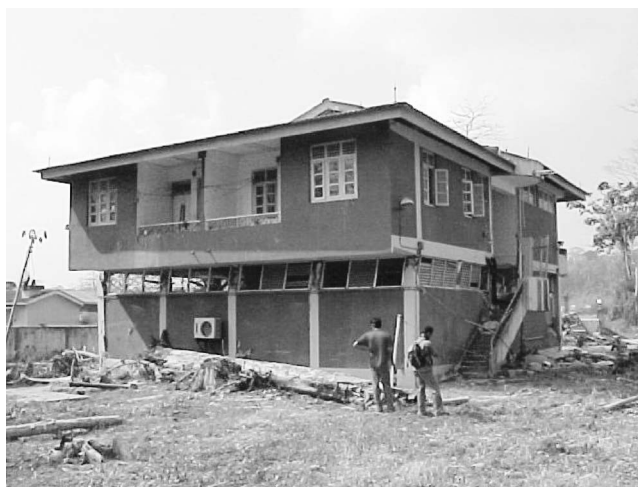
Figure 18. The BSNL telephone exchange building on higher ground at Hut Bay in Little Andaman Island was severely damaged due to earthquake shaking—it was twisted about the vertical axis during the shaking and sustained severe irreparable damage in its structural members. The structure was also flooded by the tsunami runup, and severe loss was sustained in non-structural elements and contents (photo: C. Murty).
