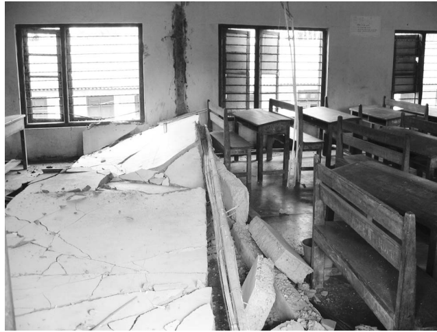
Figure 12. Slender masonry walls became dislodged because of out-of-plane instability and poor connection or no connection to the surrounding structural elements at the senior secondary school building in Adazigin, Middle Andaman Island (photo: D. Rai).
