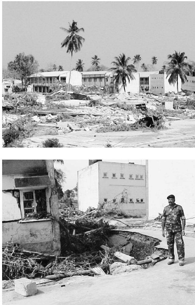
Figure 28. These buildings at the Air Force Colony in Car Nicobar Island are apparently standing after the tsunami, but their foundations have been scoured away (photos: C. Murty).
