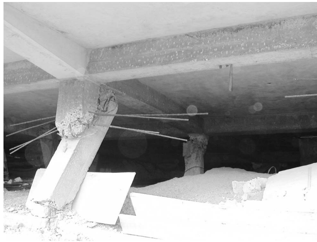
Figure 7. Buildings in Port Blair that were subjected to similar ground shaking intensity performed differently: a three-story RC-frame building collapsed in a brittle manner (photo: S. Jain).
