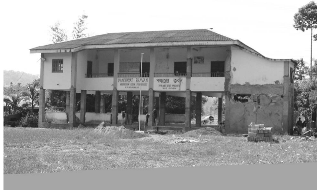
Figure 16. The Nabagram panchayat bhavan building was shaken by two earthquakes—on 14 September 2002 and 26 December 2004. Severe cracking and damage were observed in the soft first-story columns, and columns in the first story that were primarily damaged in the 2002 earthquake because of “missing” ties were now more severely damaged in the 2004 earthquake, even though they had apparently been “retrofitted” (photo: D. Rai).
