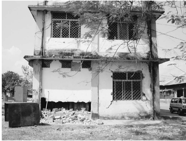
Figure 31. The old dry dock in the marine jetty dry dock complex was inundated in seawater after the event, and the masonry walls were damaged (photo: H. Kaushik).
