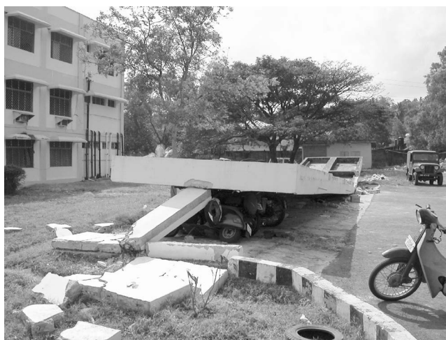
Figure 19. Collapse of a 2-m-high shelter for bicycles and motor scooters near the Port Management Board office complex in Port Blair (photo: S. Jain).
