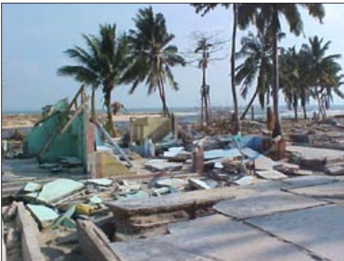
Figure 6. General destruction of built environment at Hut Bay in Little Andaman Island (photo: C.V.R. Murty).
