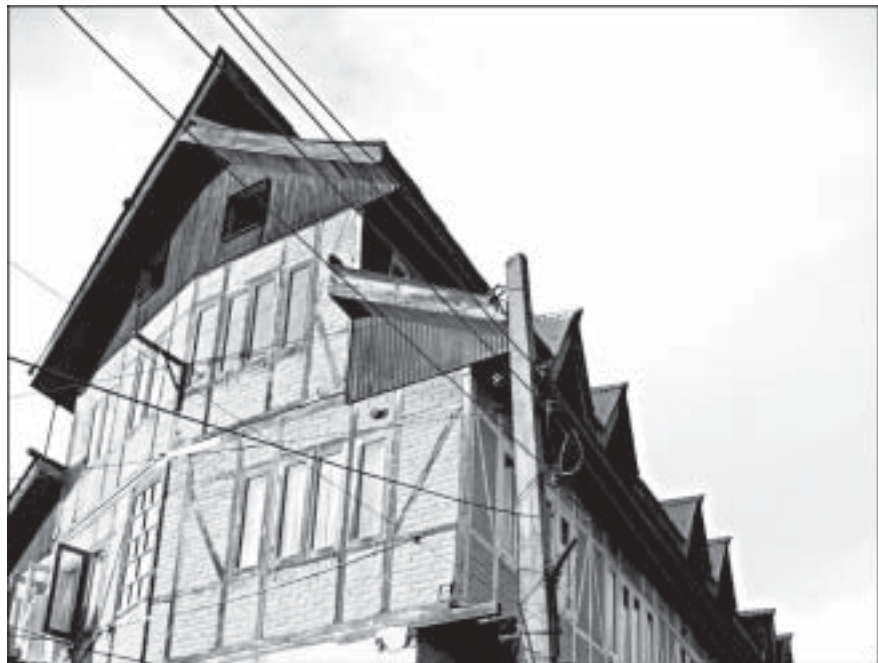
Fig 1 Dhajji-dewari system of timber-laced masonry for confining masonry in small panels withstood the earthquake without serious damage
