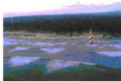
**Figure 1.** Flooding of lighthouse base due to land subsidence at Indira Point, southernmost tip of India at Great Nicobar Island. Submergence is about ~3 m caused by the *M<sub>w</sub> 9(3)* megathrust earthquake (Photo courtesy: Flight Commander Rajesh Makwana, Indian Coast Guard, Port Blair.)
