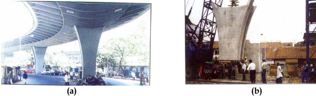
**Figure 11:** Massive Pre-cast Piers used for flyovers without disruption of underlying services and utilities: (a) JJ Hospital Flyover on Precast Piers in Delhi, and (b) Transportation of Precast Piers from site of construction to erection site (Bhattacharya, 2002)
