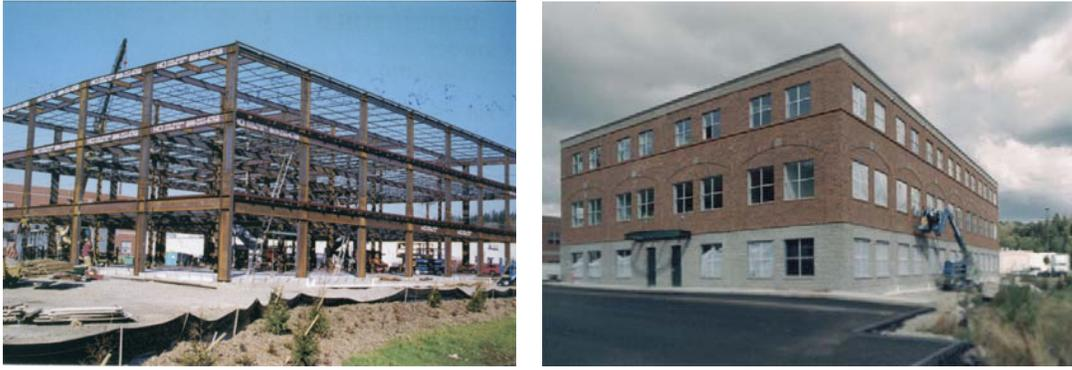
**Figure 9:** A three-storey Pre-Engineered Building under construction by assembling of pre-engineered components, and in finished state. (Source: [www.hcisteel.com](http://www.hcisteel.com), 2004)
