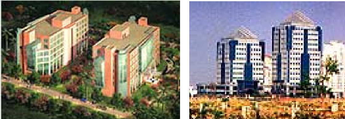
Figure 14: Large apartments and commercial complexes with captive power generating systems (Source: www.unitech-limited.com )
