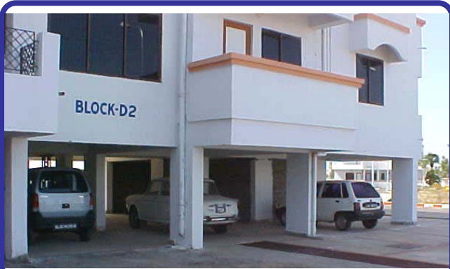
Figure 1: Ground storeys of reinforced concrete buildings are left open to facilitate parking – this is common in urban areas in India.
