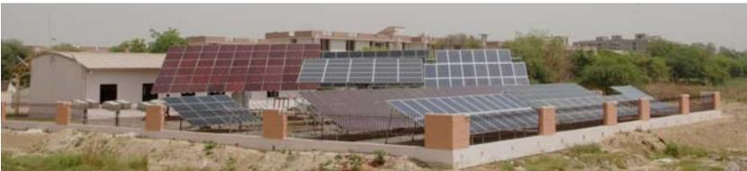
Research Enclave (SERE). Besides providing opportunity for R&D in PV technologies, the enclave acts as a demonstrator of solar based technologies. The enclave is self sufficient in its electricity needs through 5 KWp battery supported solar panels and is also feeding about 200 units/day to the IITK electricity grid.
